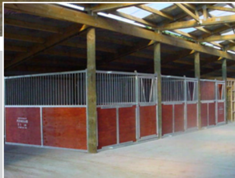
Permanent internal installation
